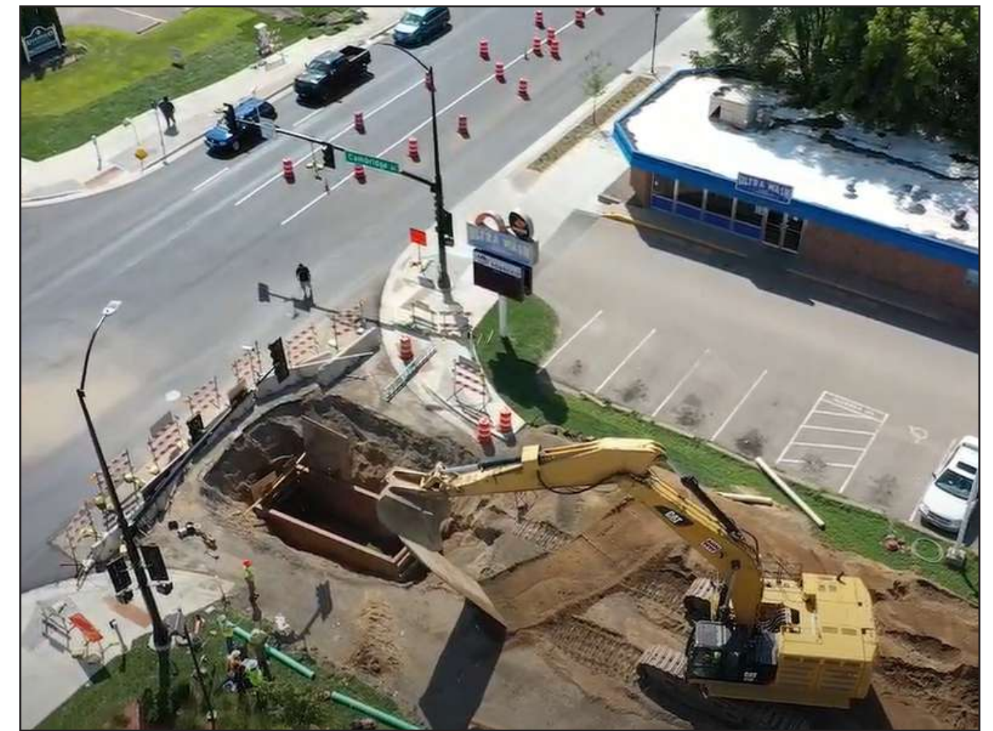
3. Replace underground utilities
