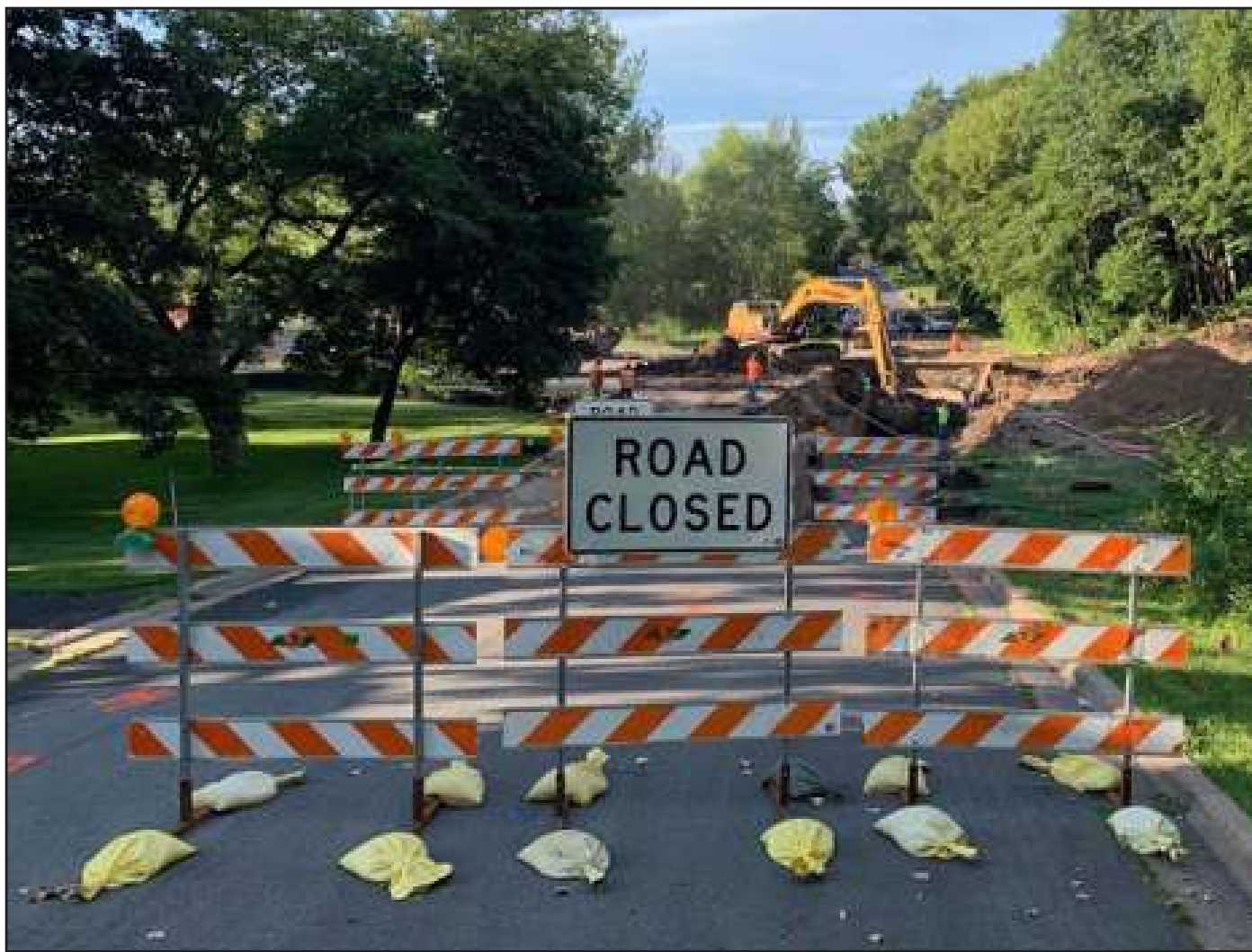
1. Place traffic control signage
