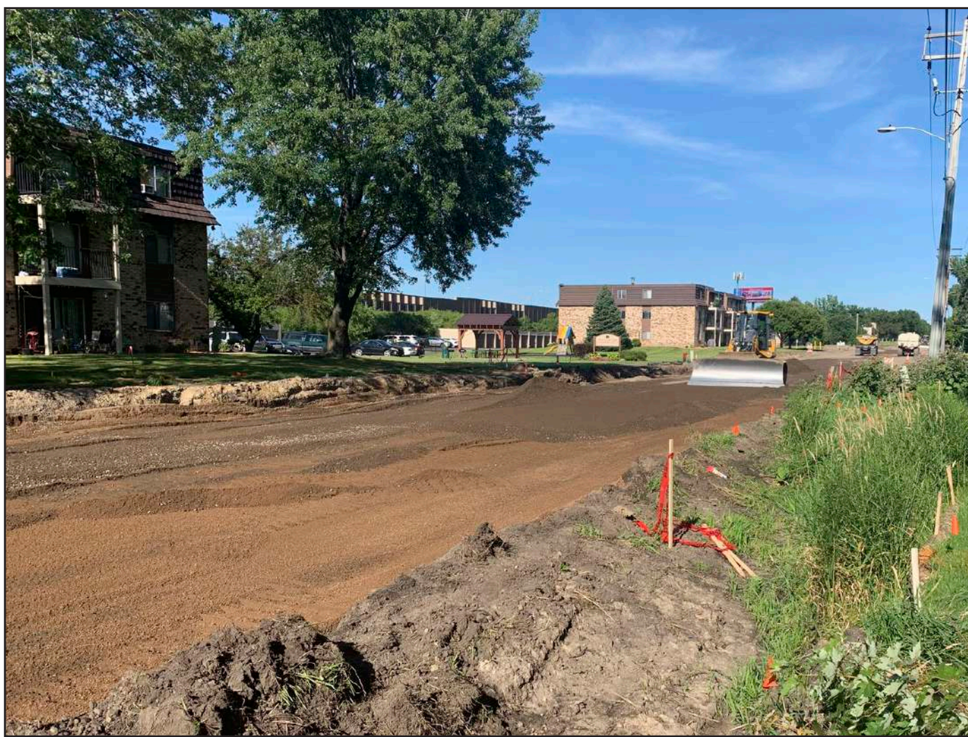
4. install new gravel/dirt base
