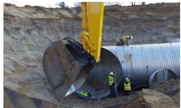
12-Foot Diameter Culvert
