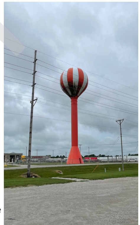
Figure 8.1 – Water Tower and Utility Lines
