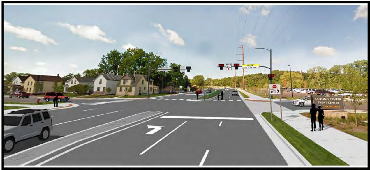
Figure 5. Overhead Pedestrian Hybrid Beacon System installed across CSAH 61 at Pine Street.
