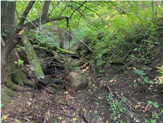
Photo 13: Erosional Feature 2 near SP-3
