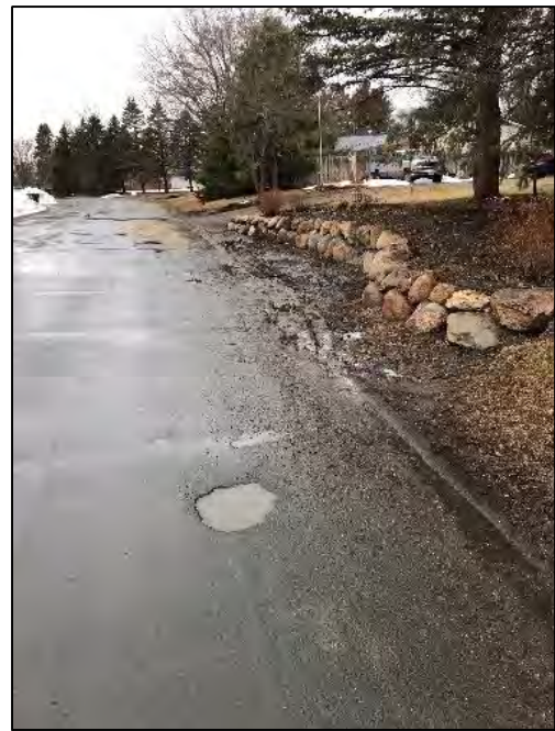
Pavement deterioration along the edges of 200 th Street
