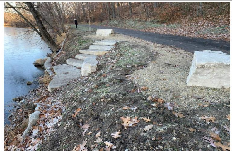
VEGETATED RIPRAP WITH LIVE STAKES
