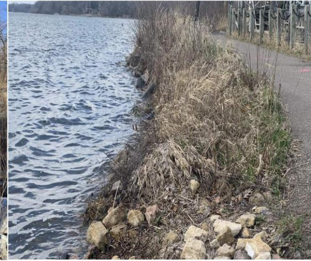
VEGETATED RIPRAP WITH LIVE STAKES
