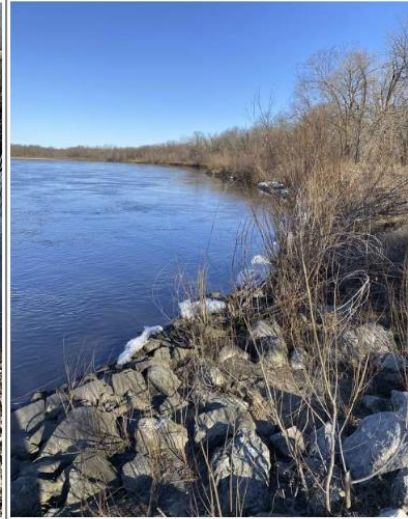
VEGETATED RIPRAP WITH LIVE STAKES
