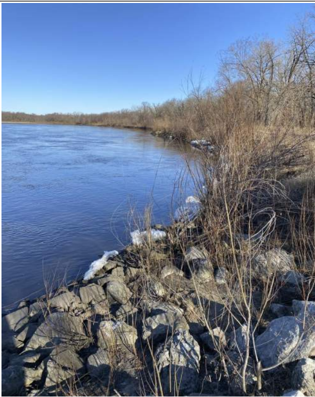
VEGETATED RIPRAP WITH LIVE STAKES
