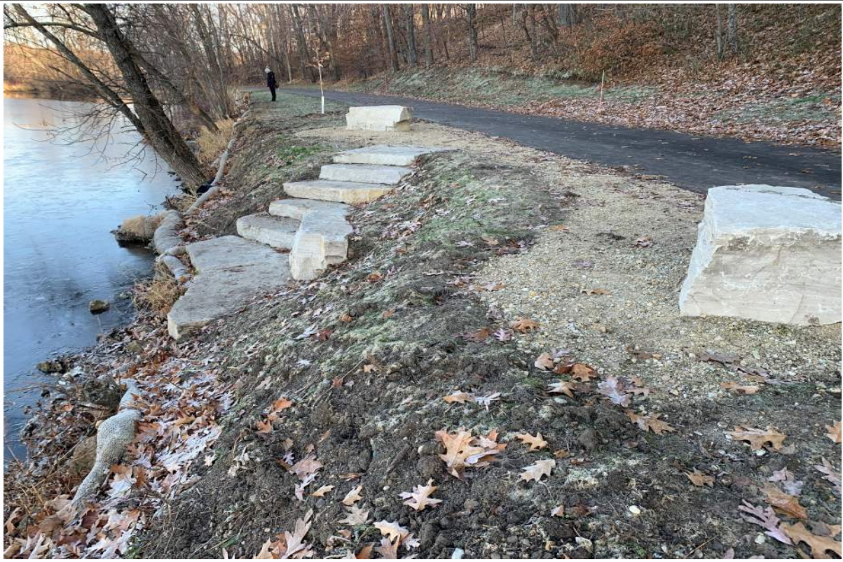
VEGETATED RIPRAP WITH LIVE STAKES
