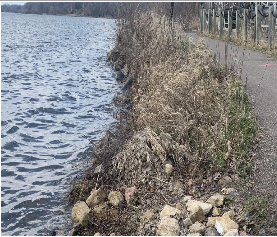
VEGETATED RIPRAP WITH LIVE STAKES
