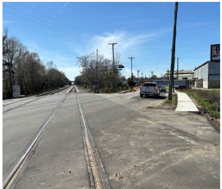
CSX RAILROAD AND SIDEWALK NEAR E LIBERTY STREET
