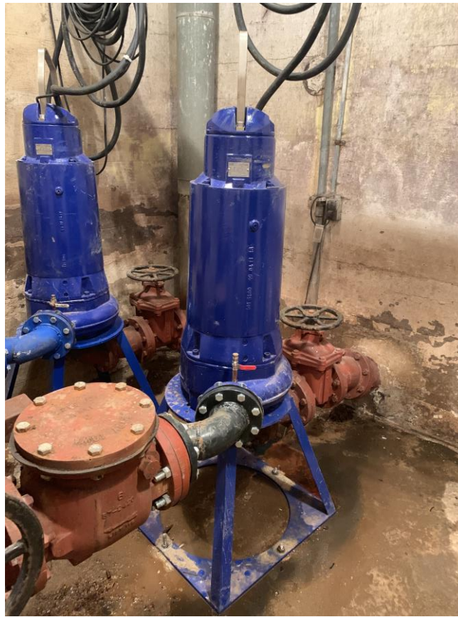
Figure 3.2 – Existing Lift Station Pumps
