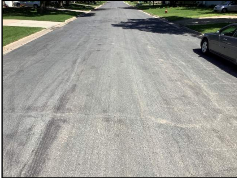
Exhibit 4 – Street Condition, 5 th Street NE
