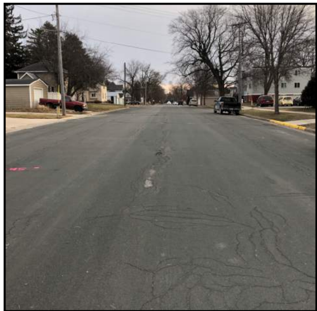
Exhibit 2 – Street Condition, 2 nd Avenue NE
