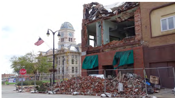
Tornado-ravaged historic building at Center Street and Main Street now demolished
