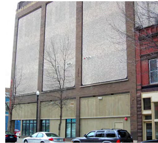
Infilling or covering over original window and door openings is prohibited in the Historic District.
