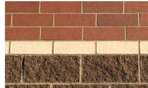
Jumbo, oversized brick and decorative concrete block are only allowed in the Central Business District.
