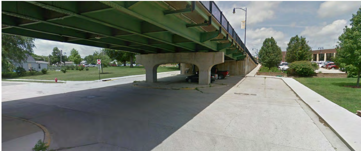
Existing conditions under the Center Street bridge
