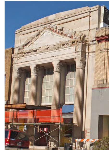
5 West Main Street undergoing renovation
