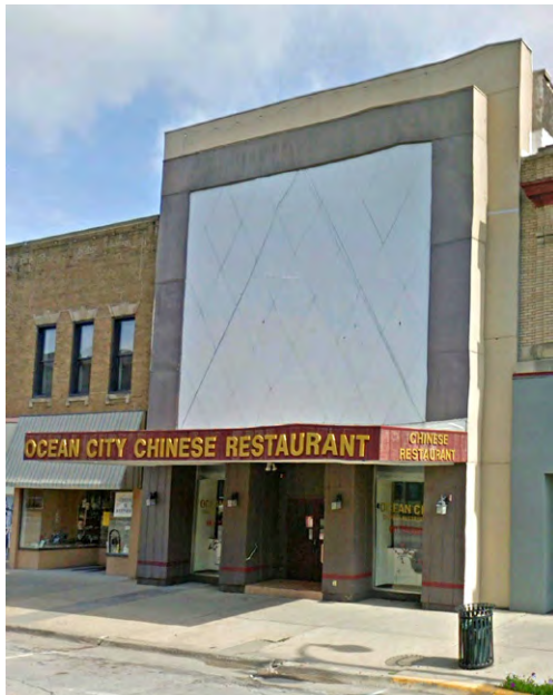
5 West Main Street before renovation
