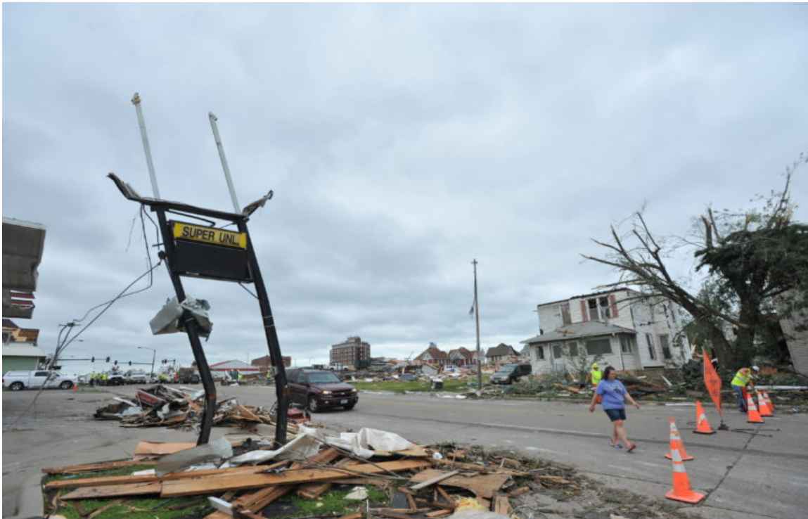
Figure 1: Damage to businesses and homes on Highway 14 in the aftermath of the July 2018 tornado
