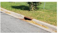
Roadways are almost always 'crowned' meaning the center of the roadway is higher than the roadway edges. It is therefore the duty of the roadway edges to convey/transport water from the street to either a ditch system or a storm sewer inlet.
