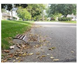
some amount of curb at inlets would be required for compatibility with storm drainage inlets.
