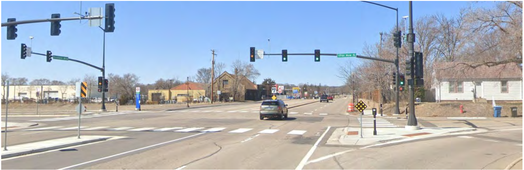
Existing intersection at Excelsior Boulevard & 17 th Avenue
