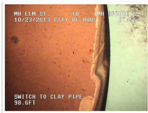
Exhibit 9 – End Sanitary Sewer Main Repair 100-ft North of Elm Street
