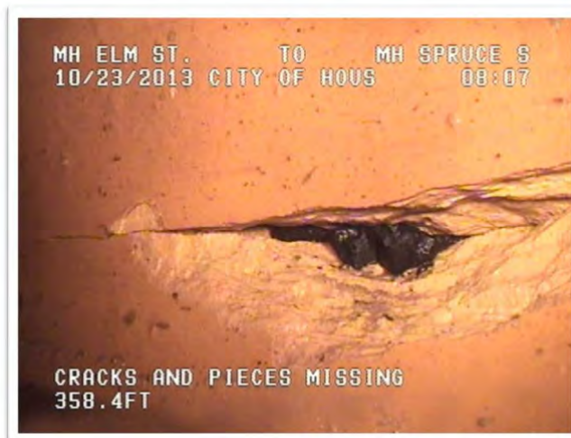
Exhibit 10 – Damaged Clay Pipe Sanitary Sewer Main 20-ft South of Spruce Street
