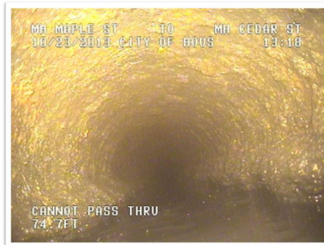
Exhibit 7 – Cast Iron Sanitary Sewer Main Obstructed 75-ft North of Maple Street
