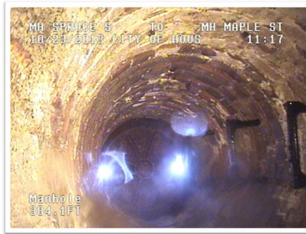
Exhibit 8 – Brick Sanitary Sewer Manhole Main at Maple Street
