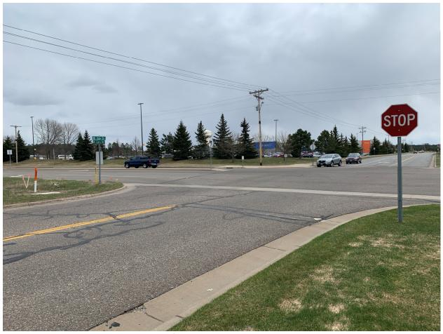
Figure 3: Isle Drive Lane Configuration with Valley Gutter within the intersection
