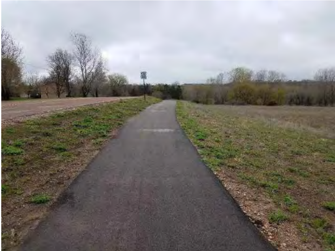
Trail to south of roadway and slope. Facing east.
