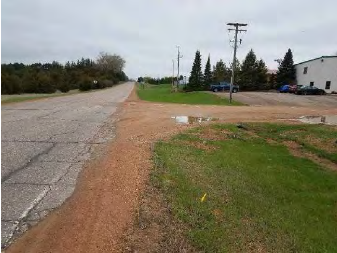
East side of roadway R/W, demonstrating utilities/grading. Facing west.
