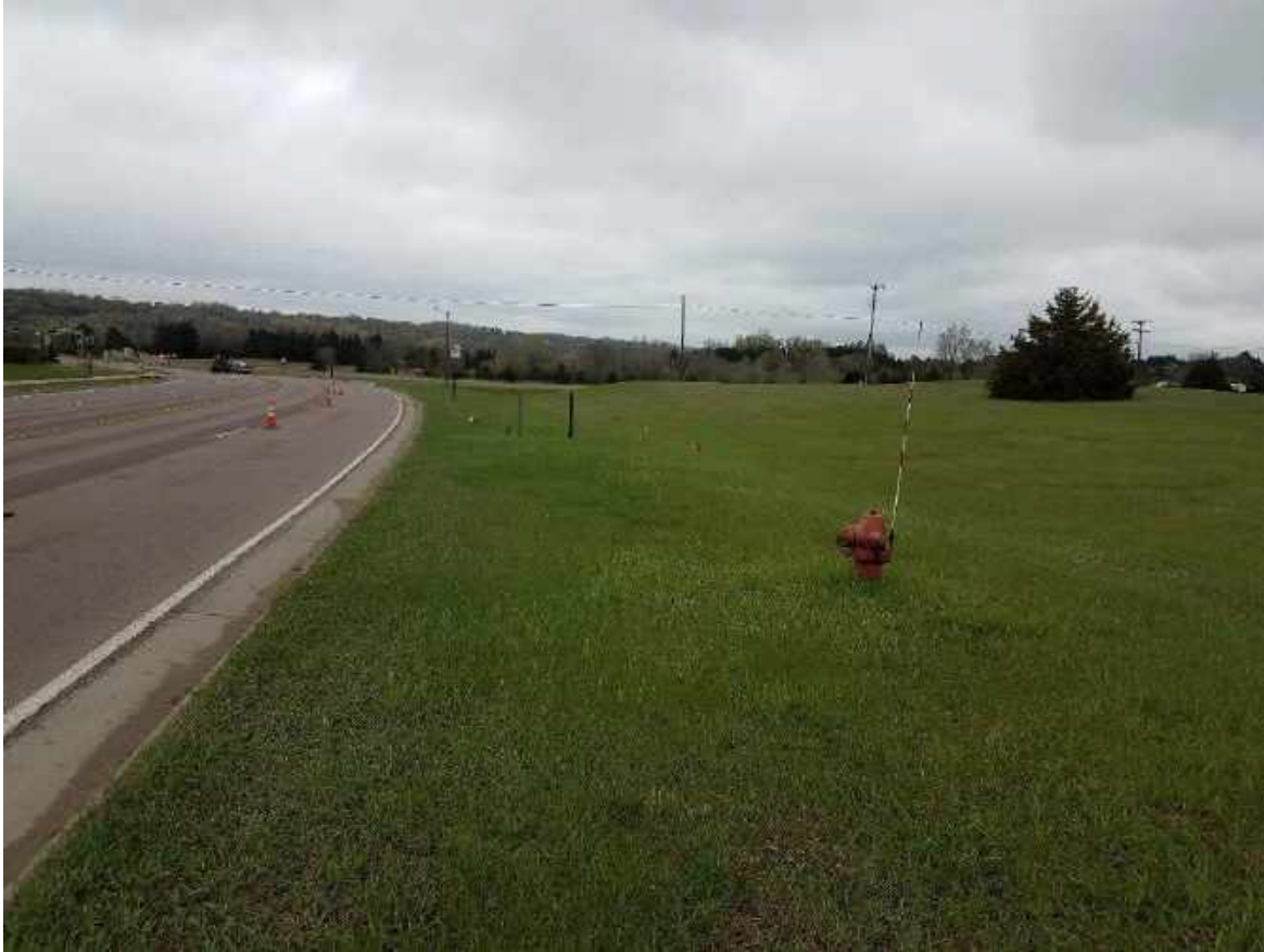
North of 190 th Street W, west side of roadway R/W, demonstrating utilities/grading. Facing south.
