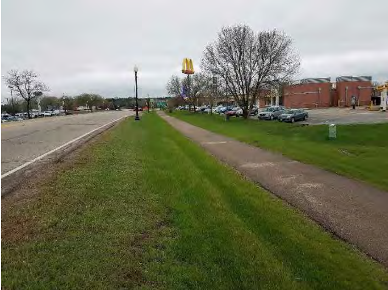
View to the northwest along 2 nd Street W (TH 282), showing trail and ditch.
