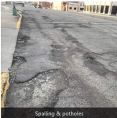
Spalling & potholes
