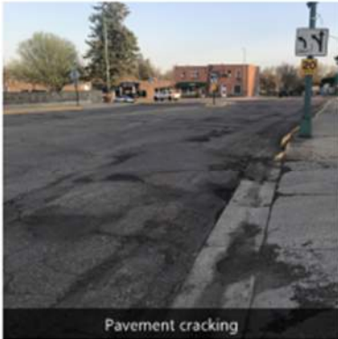
Pavement cracking
