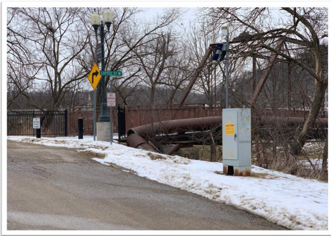
Exhibit 9 – Utility Condition, Watermain attached to Historic Bridge
