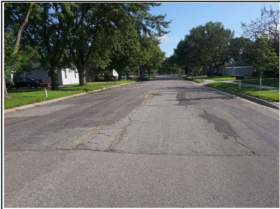
Looking Northerly along N 4th Street near N 5th Street
