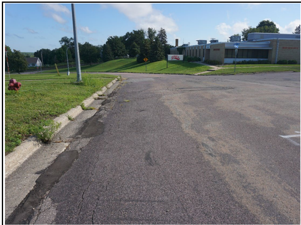
Looking Northerly along N 4th Street near Peck Street
