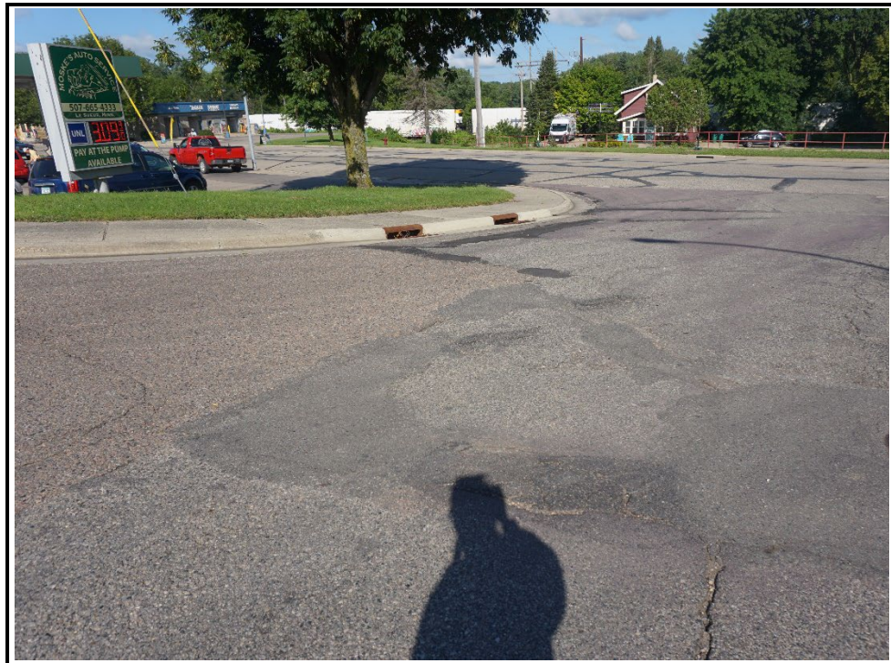
Looking Southwesterly at Cathcart Street and Commerce Street Intersection
