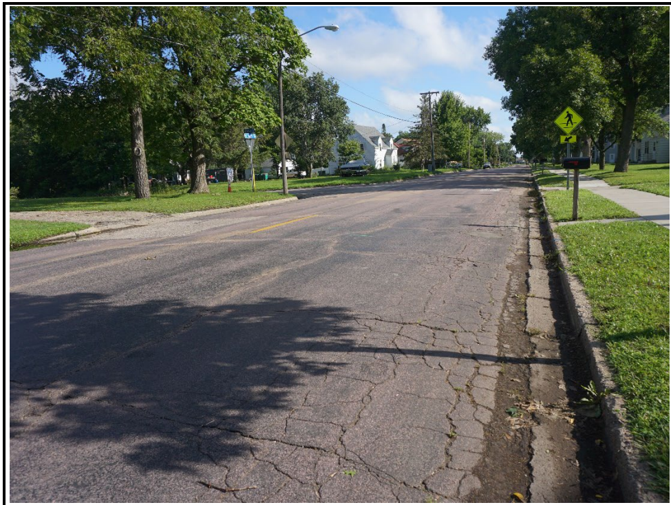
Looking Northerly along N 4th Street near Grove Street
