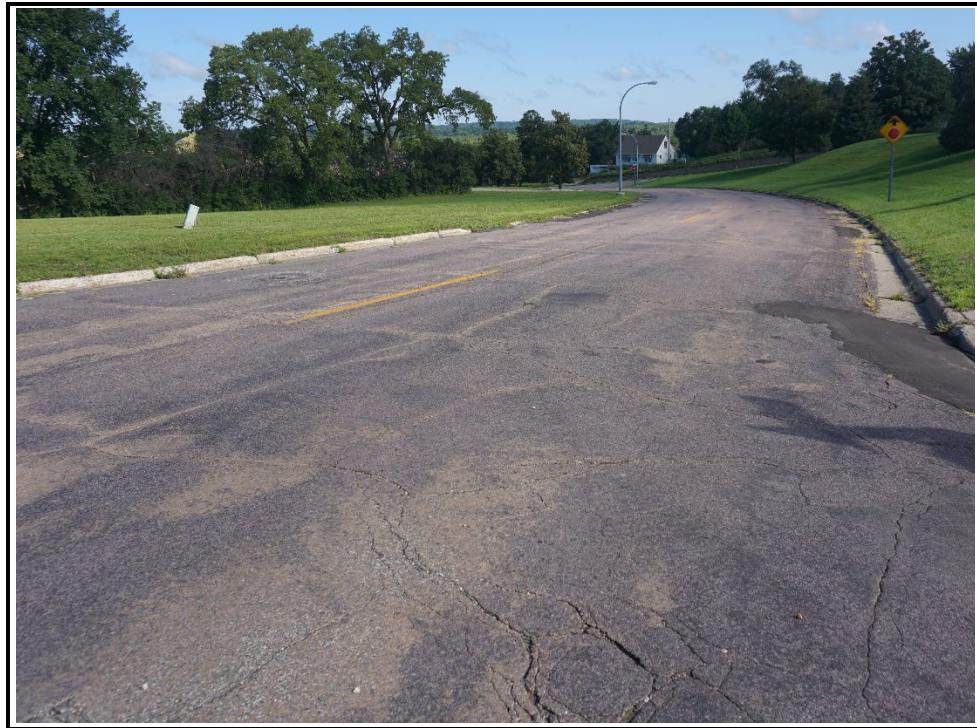
Looking Northwesterly along N 4th Street at Peck Street
