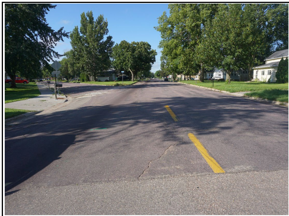
Looking Southerly along N 4th Street near N 5th Street
