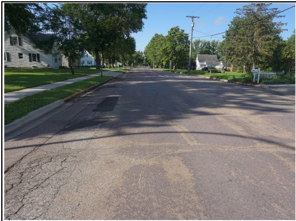
Looking Southerly along N 4th Street near Grove Street
