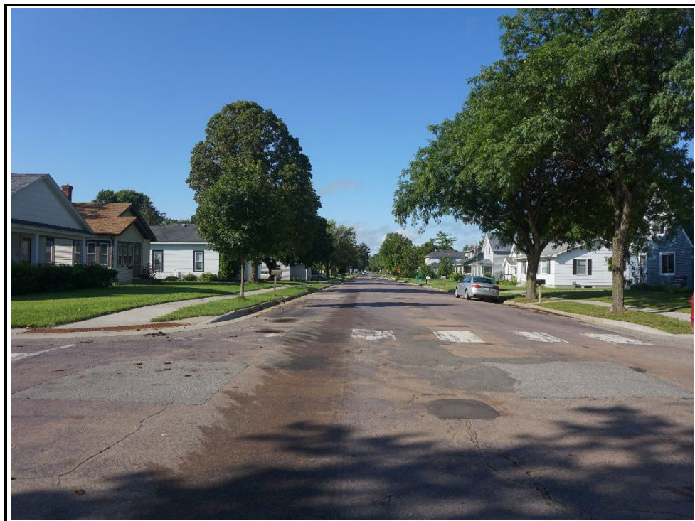
Looking Southerly along N 4th Street at Swan Street
