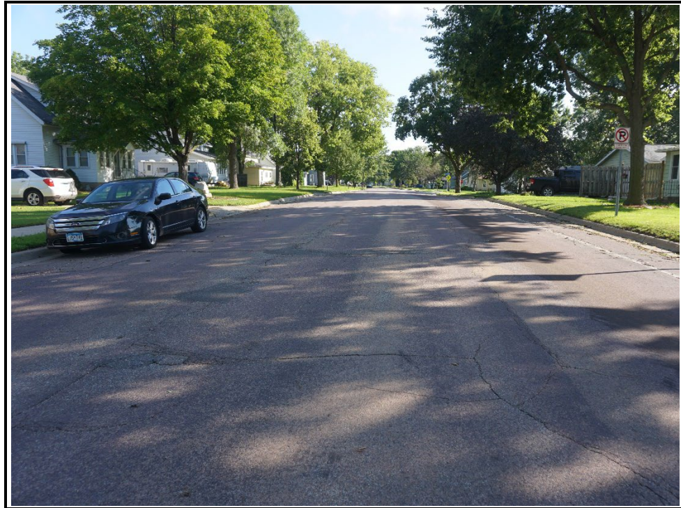
Looking Northerly along N 4th Street at Oak Street
