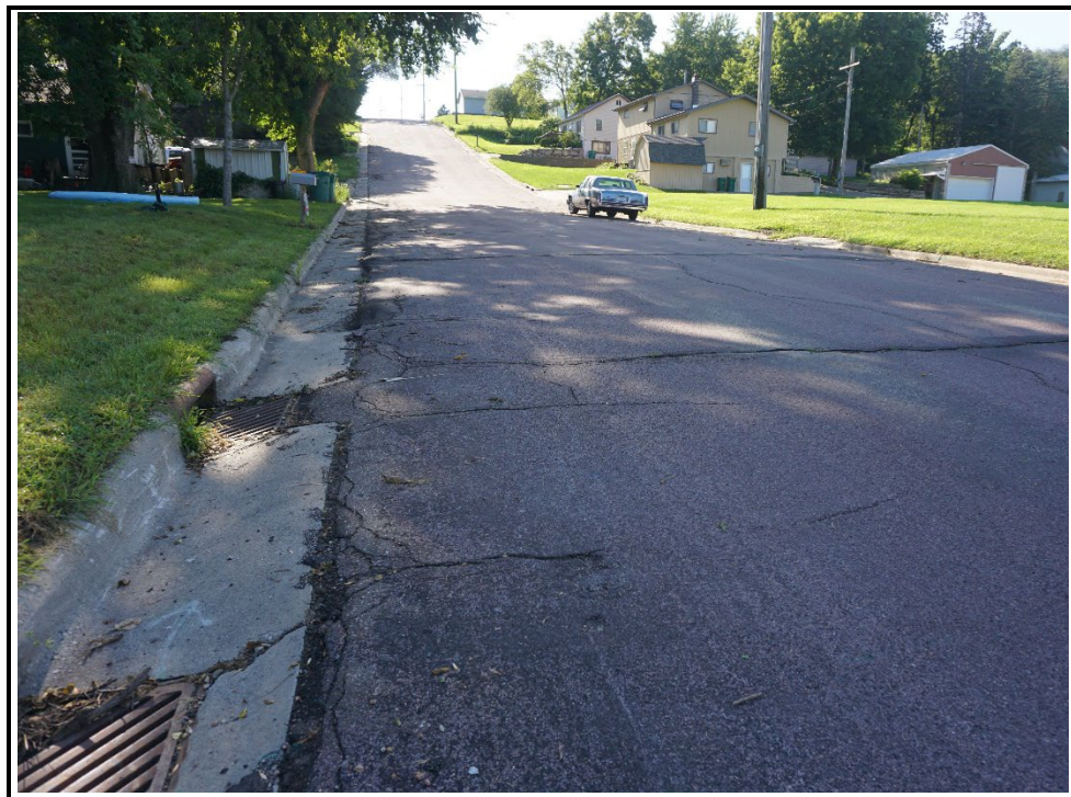
Looking Easterly along Cathcart Street near Commerce Street
