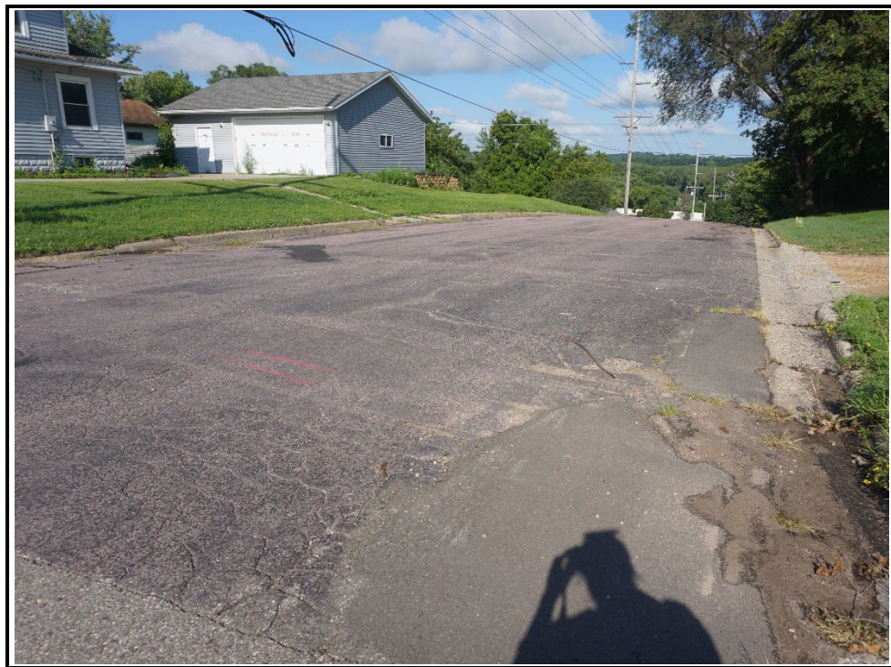
Looking Westerly along Cathcart Street at N 4th Street
