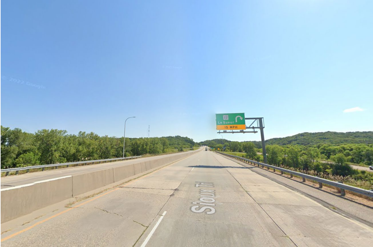
Highway 169 Interchange with CSAH 22, facing North
