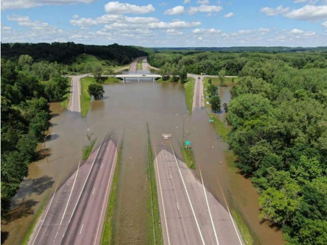
Flooding at the Southern Extent of the Project Area – Highway 169 and MN Highway 93
