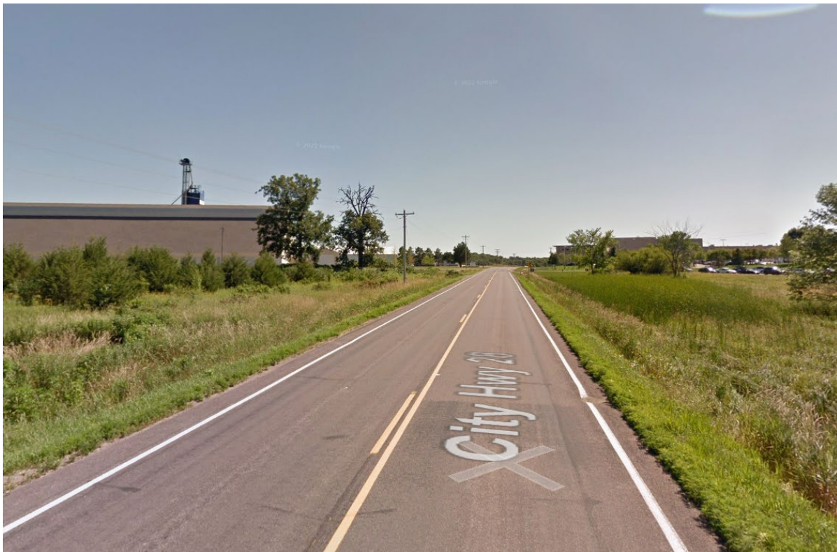
CSAH 28 in front of the Cambria Plant and Processing Facility, facing South
