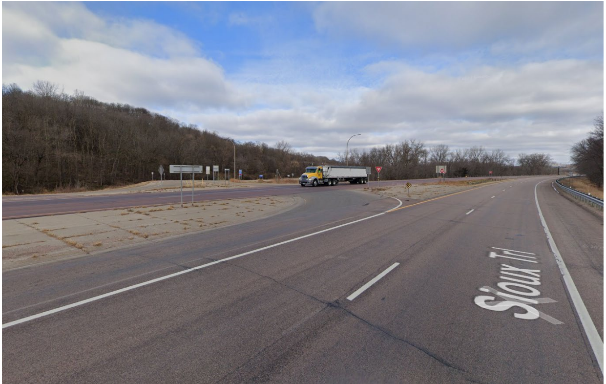
Intersection with MN Highway 93 (northern intersection)
