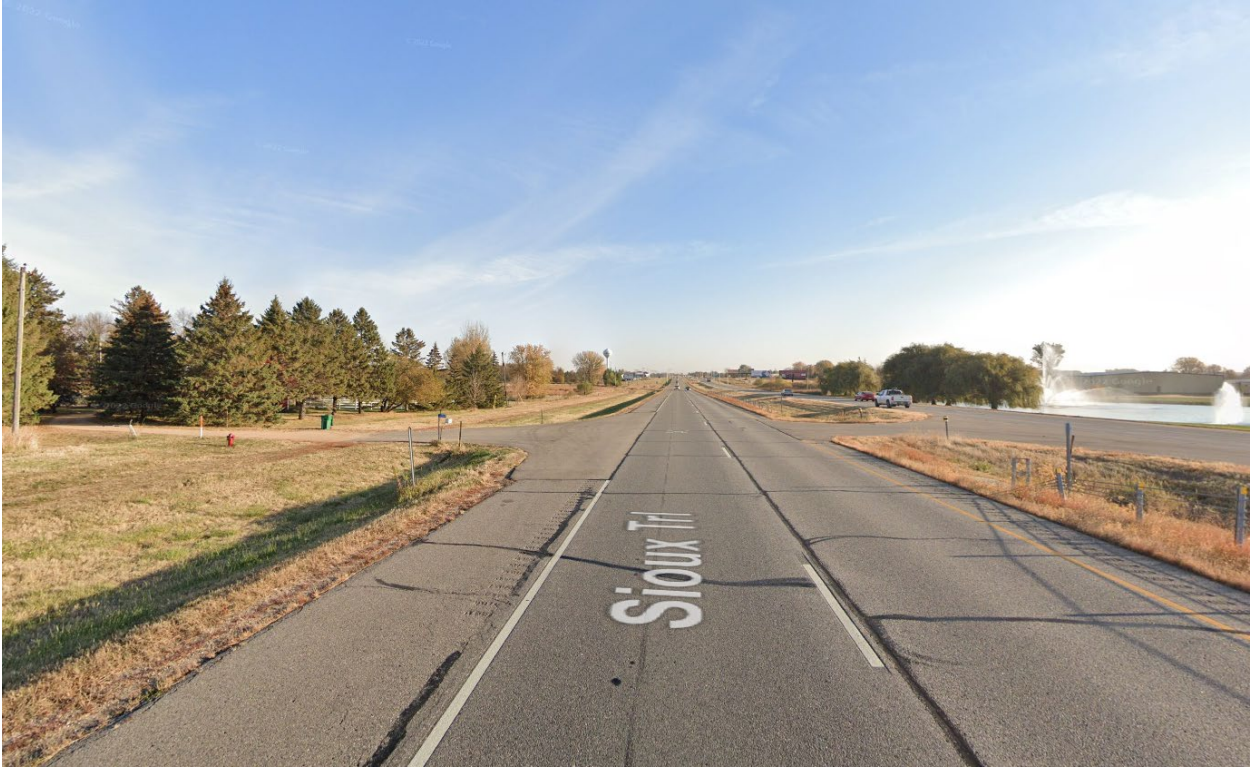
Private Driveway Access (1) off of Highway 169, facing North
