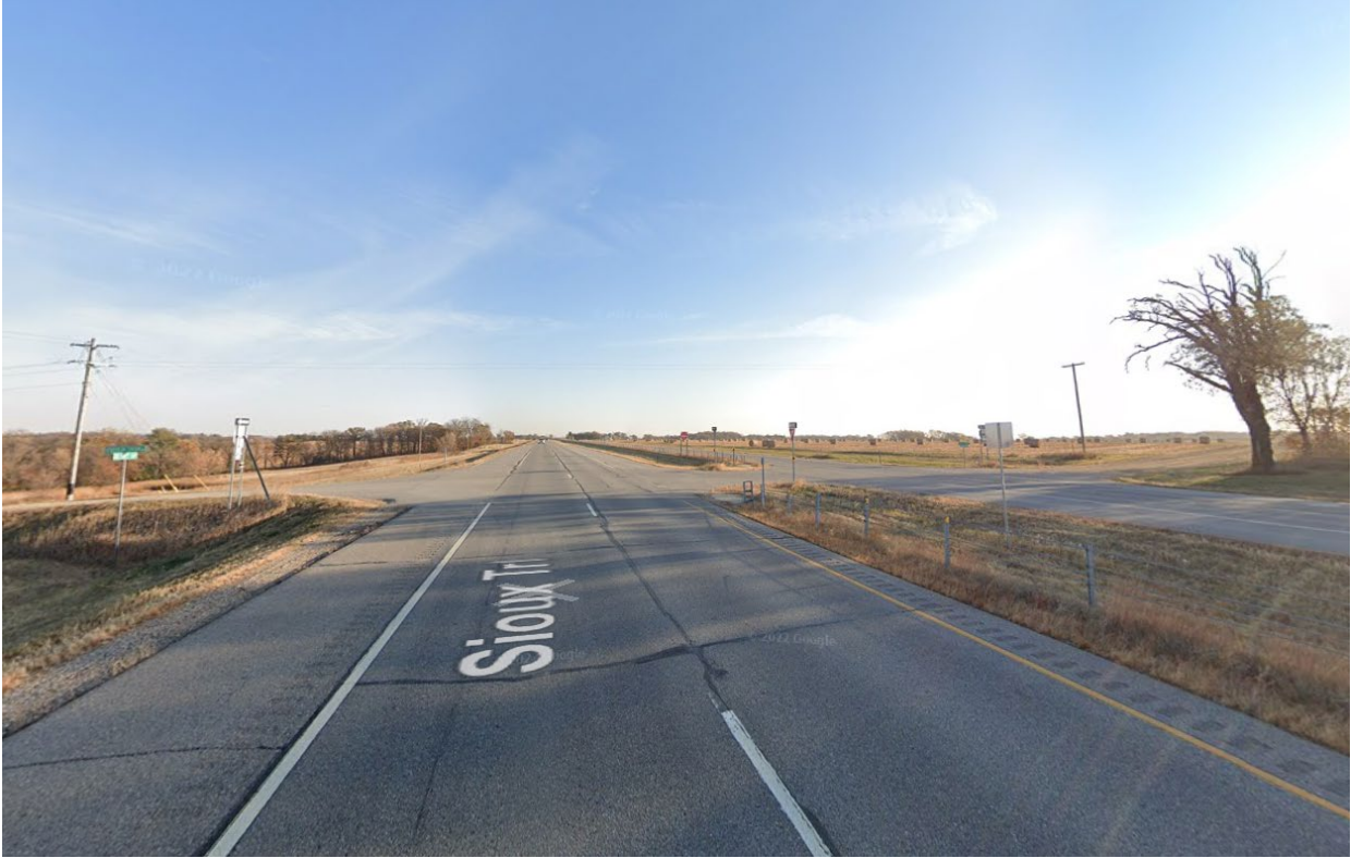
Highway 169 Intersection with Henderson Station Road, facing North (Northern Project Extent)
