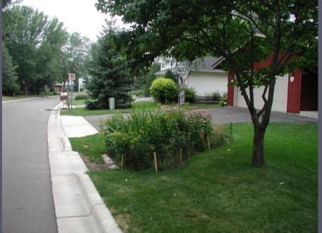
Shallow depression behind the curb designed to accept runoff from the street and infiltrate it.
