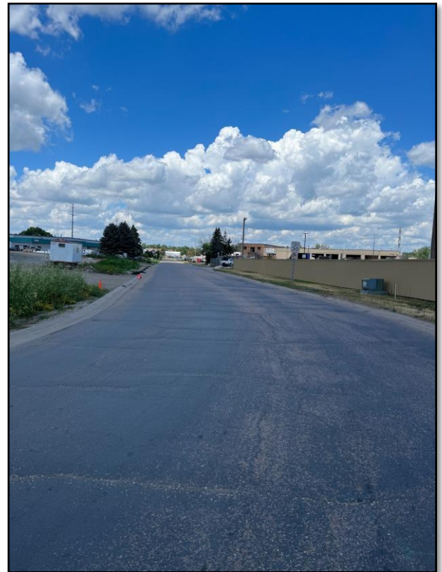
Exhibit 3 - Existing Spruce Street
