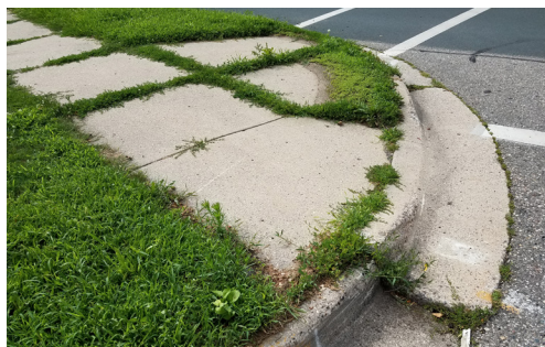
A non-compliant pedestrian ramp with vertical discontinuities greater than 1/2 inch, vegetation growing through cracks, and no detectable warning such as truncated domes.
