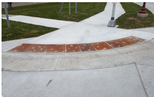
An ADA-compliant, blended transition or fan, pedestrian ramp with truncated domes and easy access to the pedestrian access route.
