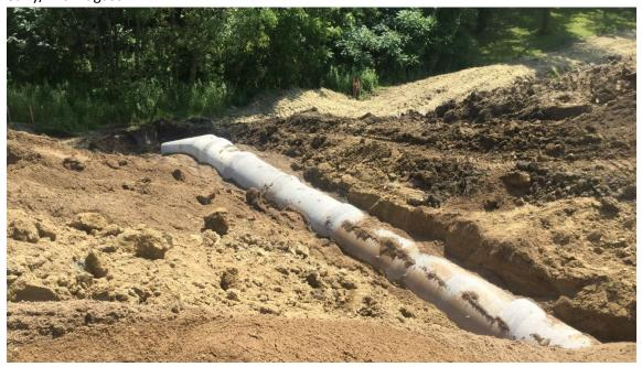
The picture above shows a storm sewer pipe being installed near Fairlawn in a 28-foot deep trench.
