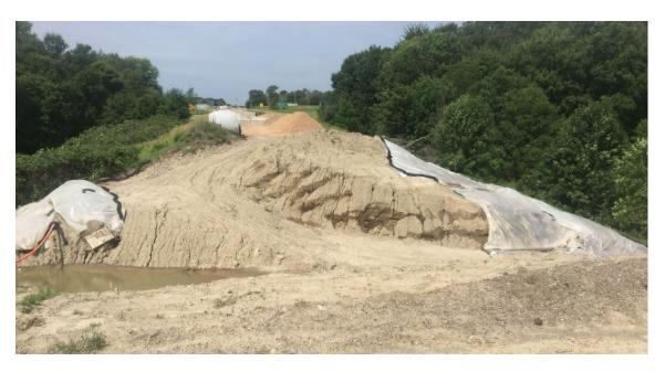
The picture above shows the 35-foot deep trench where the 6-foot pipe will be installed.
