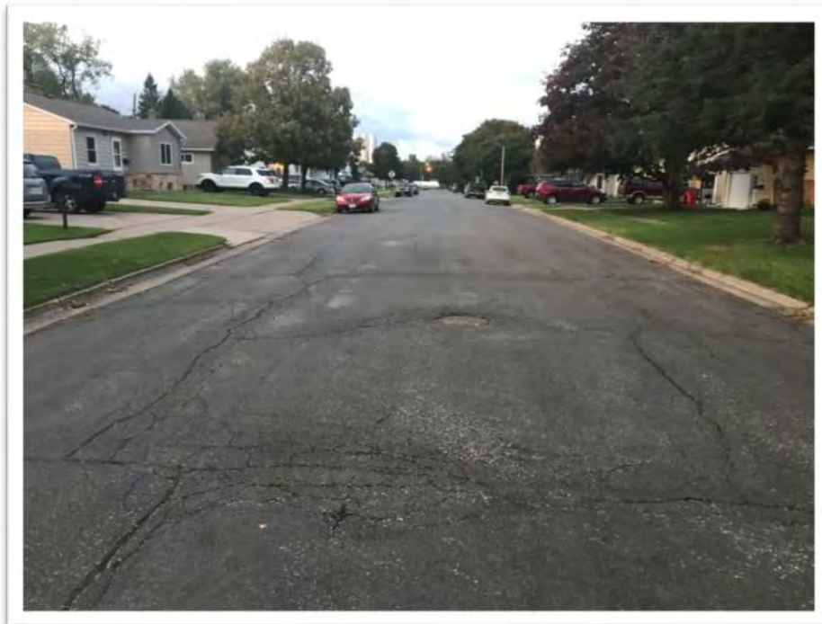
Exhibit 4 – Pavement Condition, 2 nd Street Southwest
