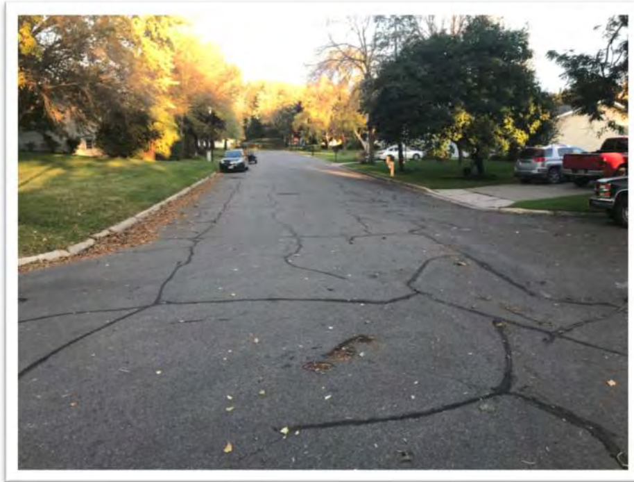
Exhibit 1 – Street & Curb Condition, Hillcrest Second Addition
