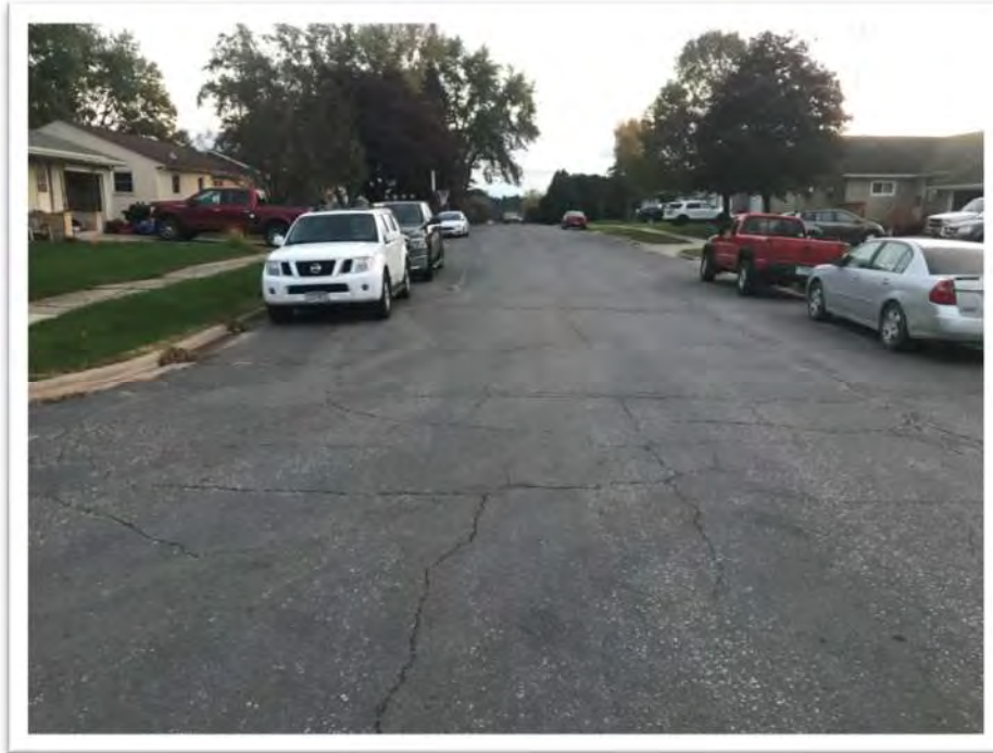
Exhibit 3 – Pavement Condition, 2 nd Street Southwest
