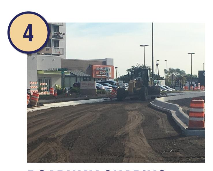
**ROADWAY SHAPING** Gravel base is compacted in preparation for paving.
