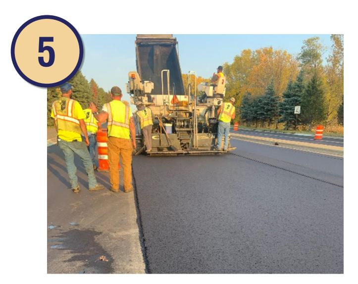
**ROADWAY PAVING** Paving occurs in two layers.
