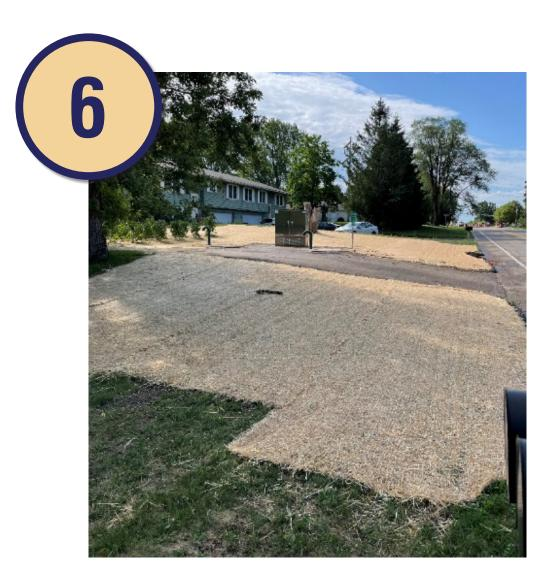
**RESTORATION** Grass that is disturbed during construction is restored with seed and erosion control blanket.
