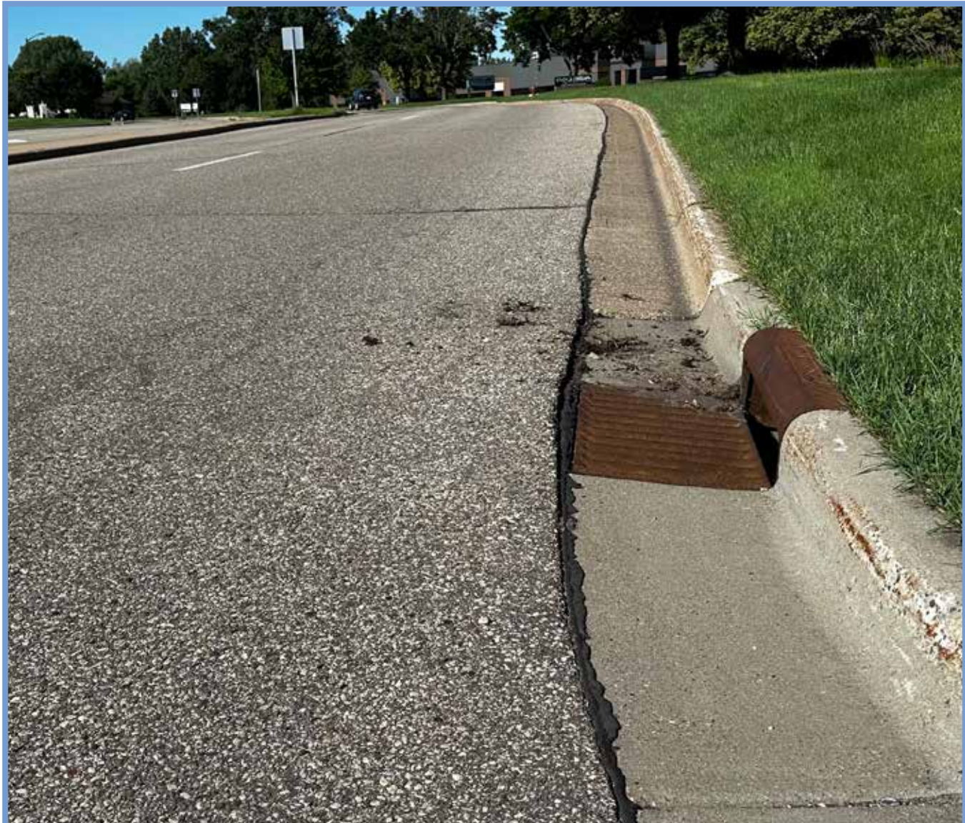
CITY STANDARD BARRIER (B618) CURB
