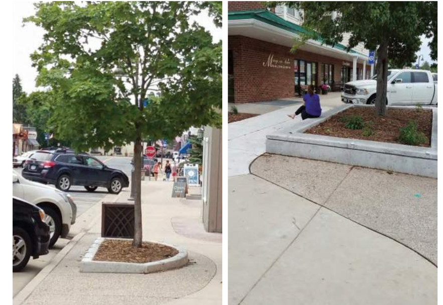
Planter Curbs & Walls
