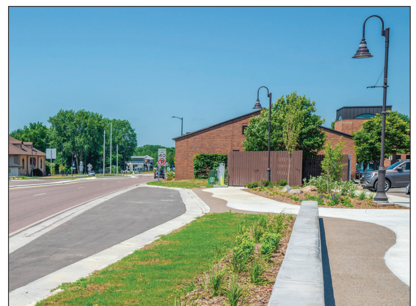
9. Turf restoration, signage, and striping
