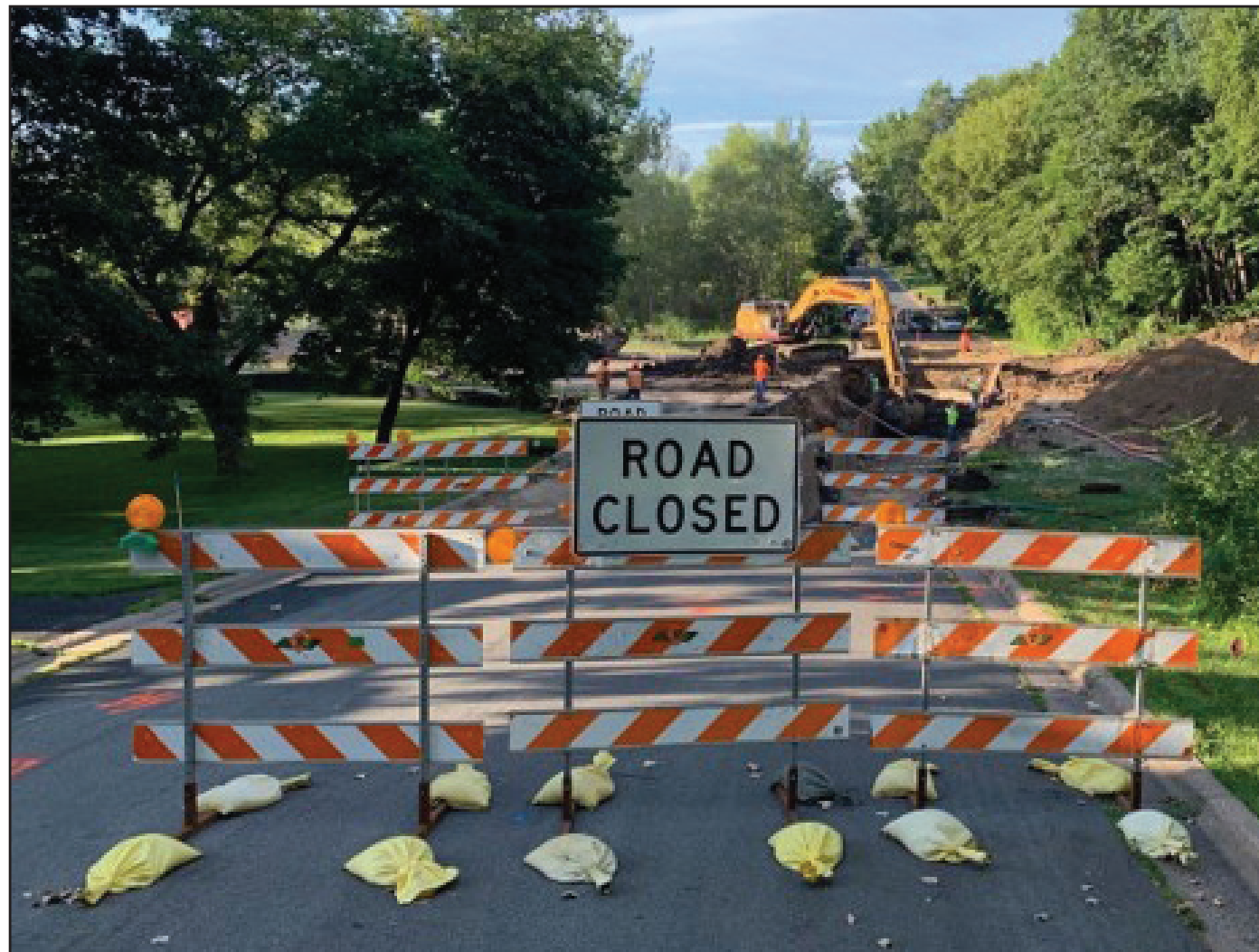
1. Place traffic control signage
