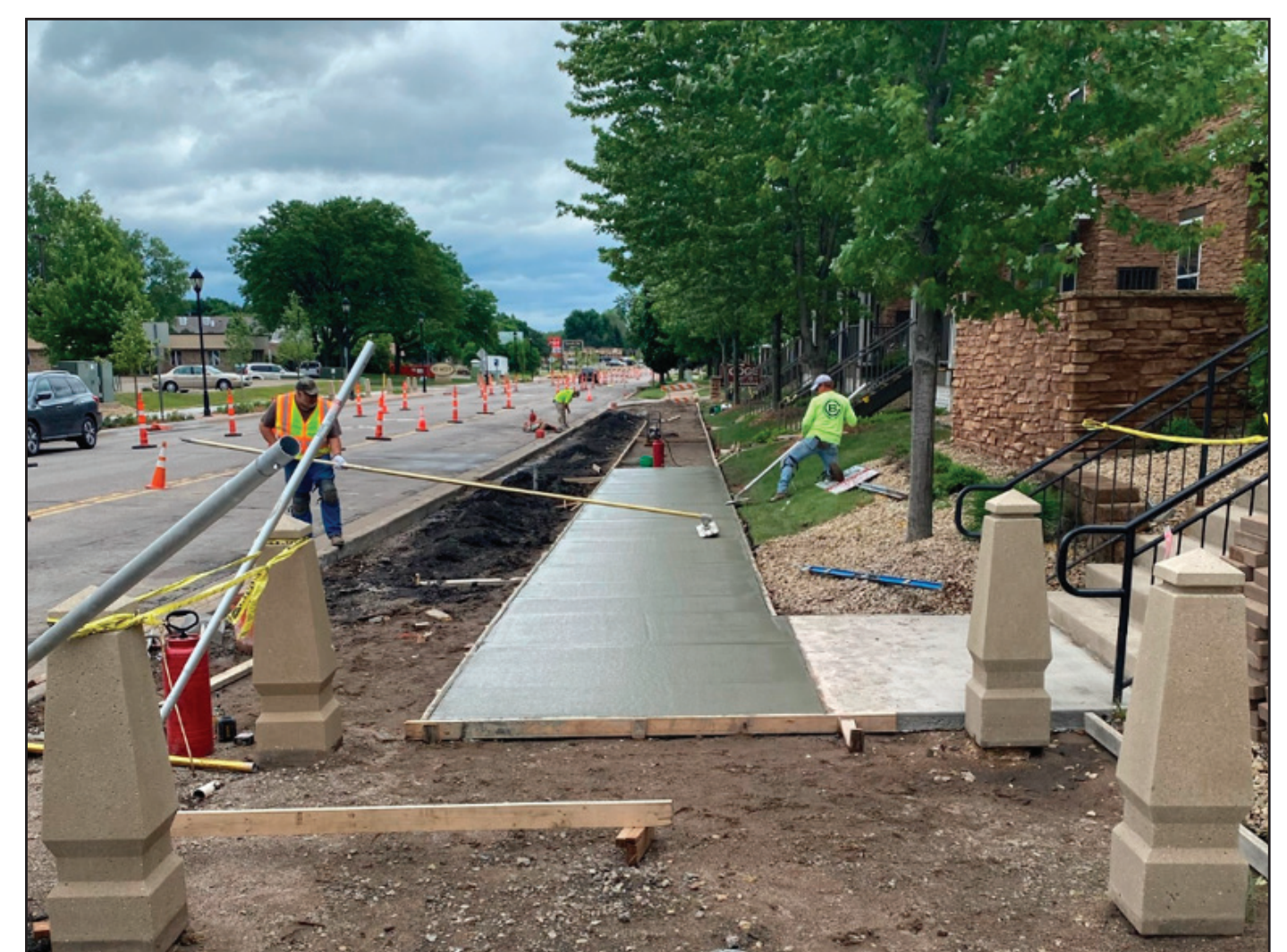
6. Install sidewalks, trails, and driveways
