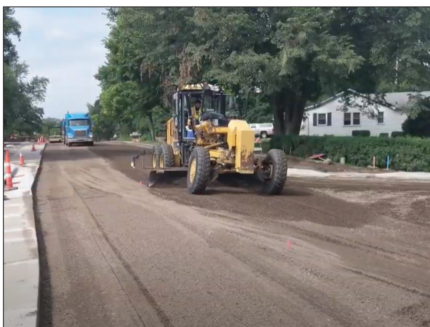
7. Grade road base
