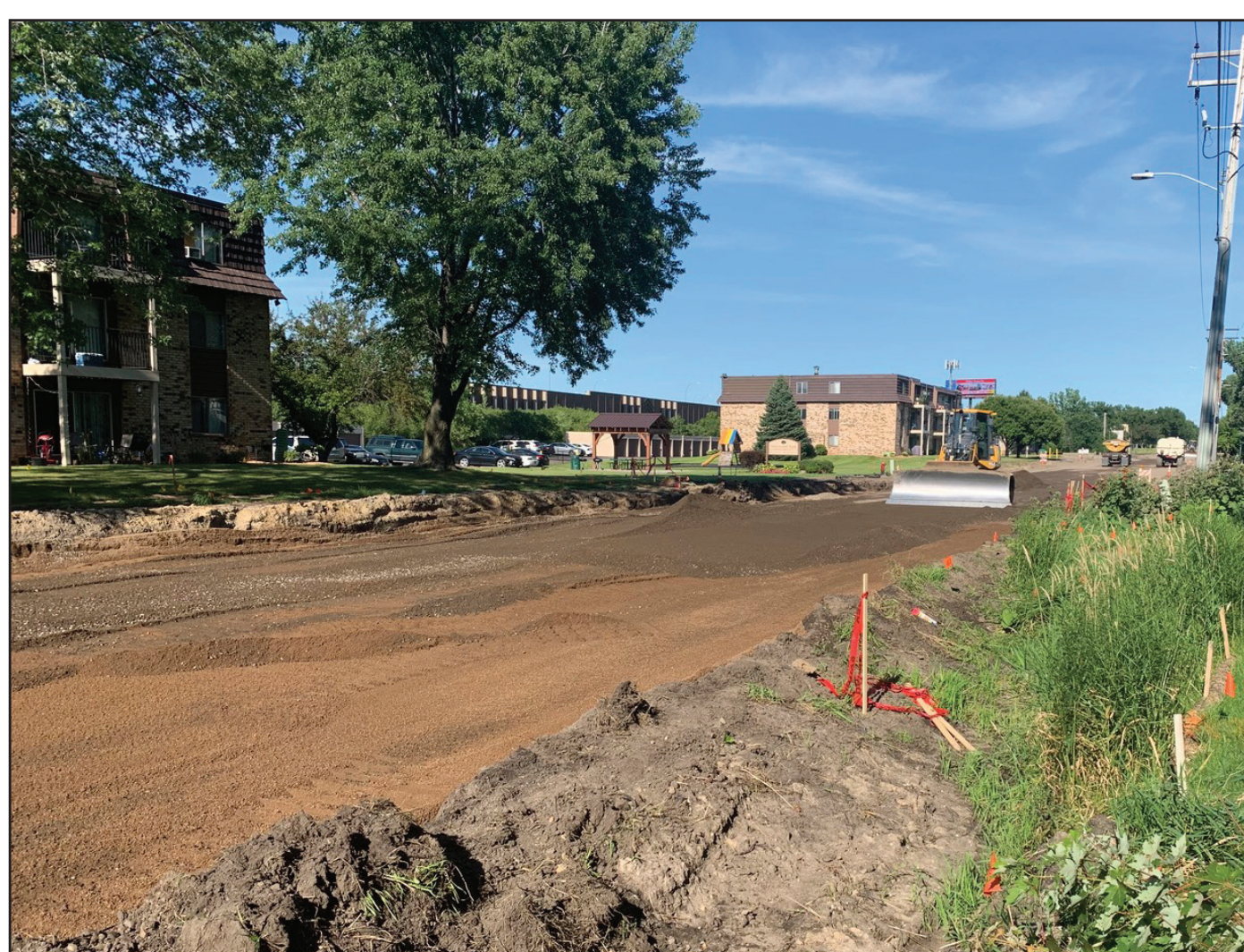
4. install new gravel base
