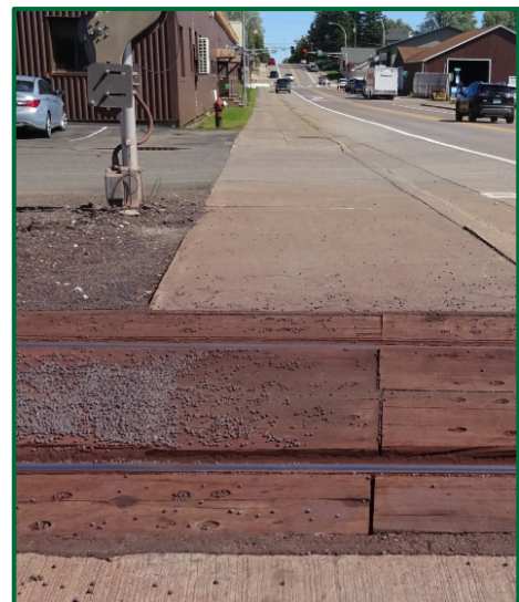
Taconite pellets dropped from trains are hazardous for pedestrians walking on 2 nd Street sidewalks.
