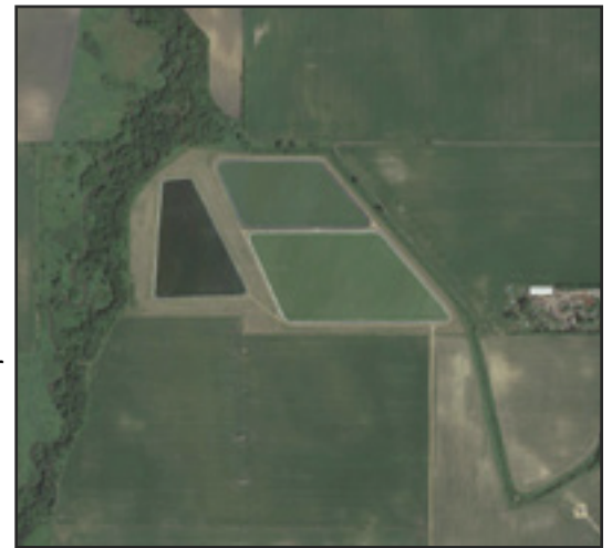
Stabilization pond system outside the City of Elmore
