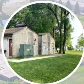
WASTEWATER INFRASTRUCTURE MITIGATION
