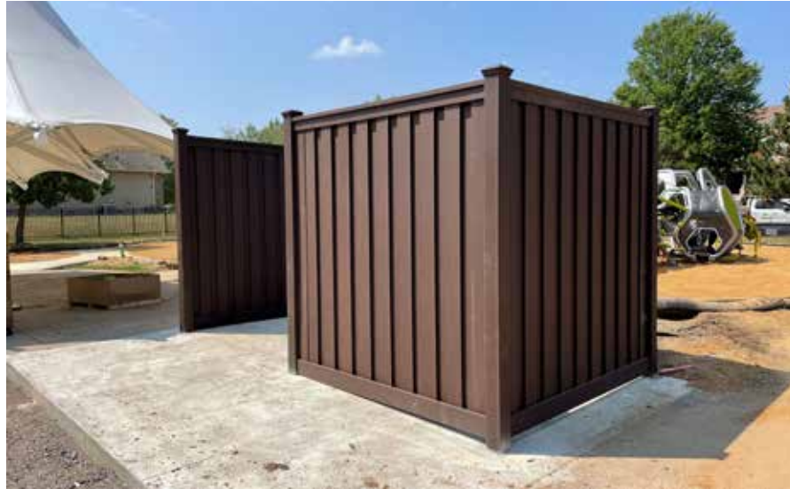
BASE LEVEL RESTROOM (PORTABLE TOILET ENCLOSURE): 8' X 16'
