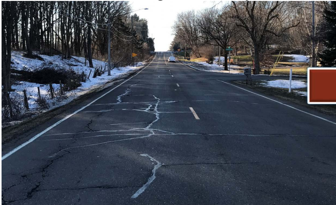
Existing Rural Roadway
