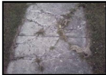
Cracking
