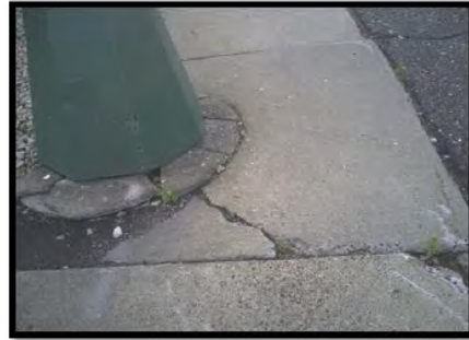
Traffic Signal Pole
