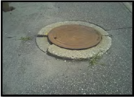
Traffic Signal Handhole
