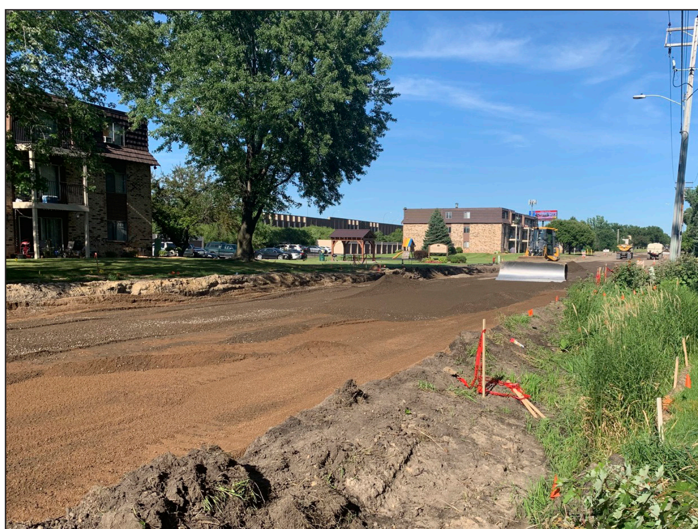
4. install new gravel base
