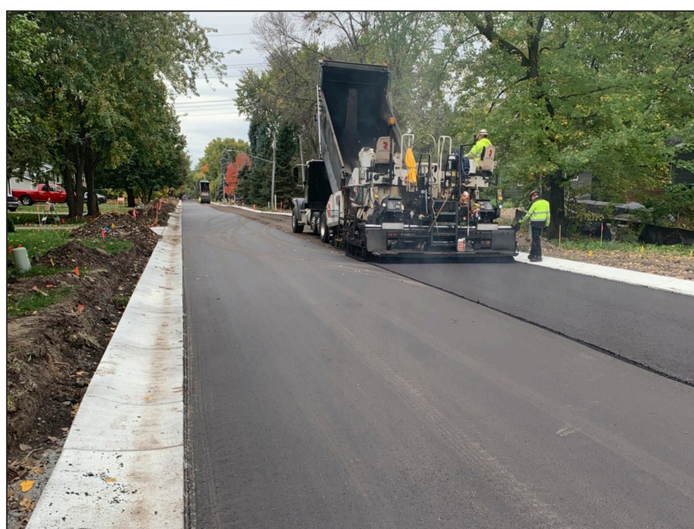
8. Pave the roadway (more than one layer)
