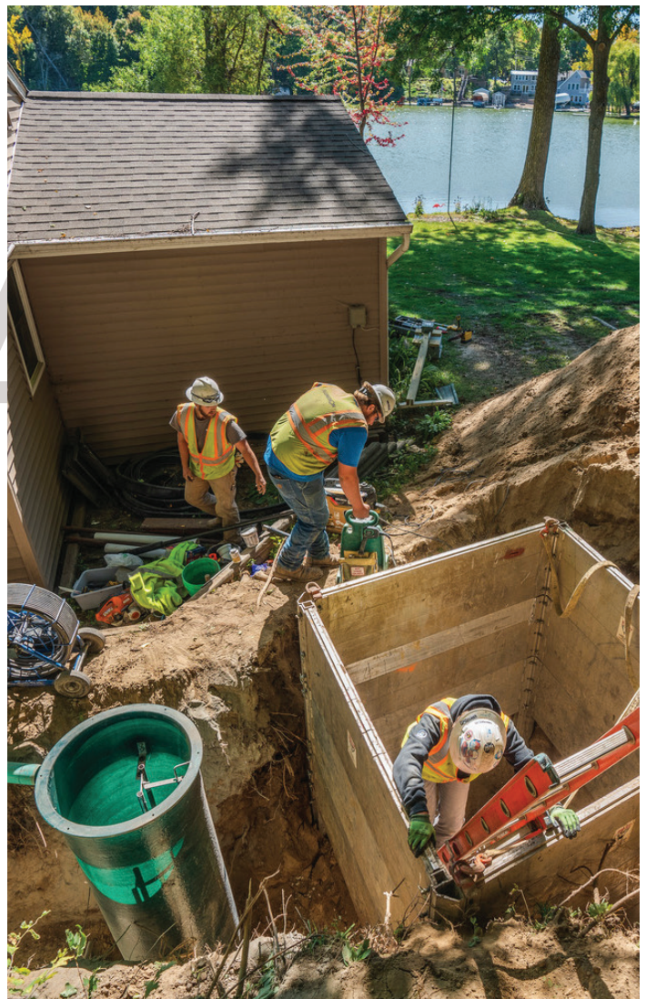
West Jefferson Sewer Construction
