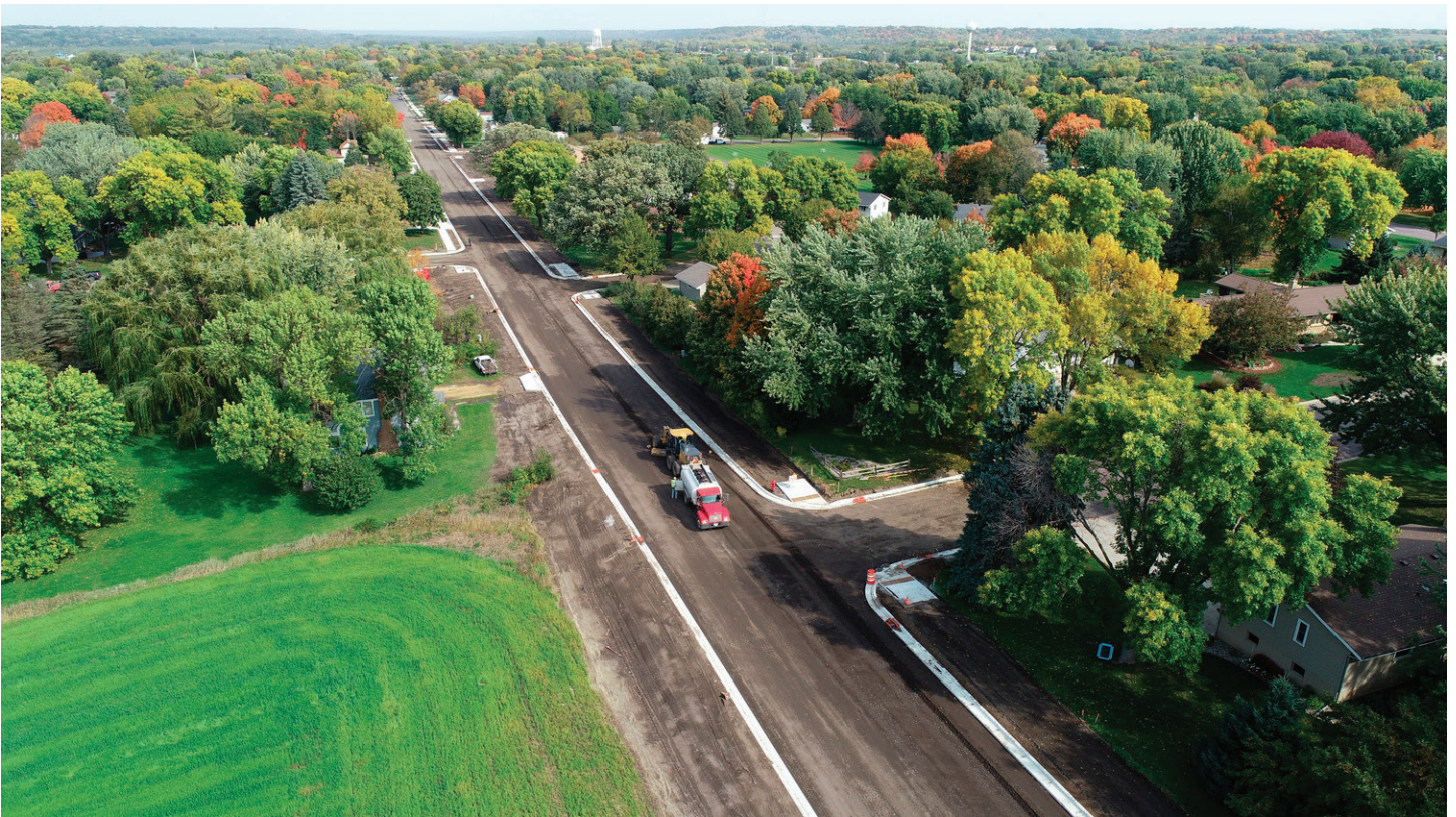
Trunk Highway 112 Turnback Construction
