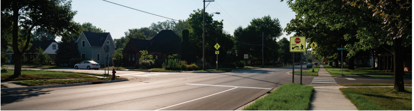
T.A.P. Sidewalk Project
